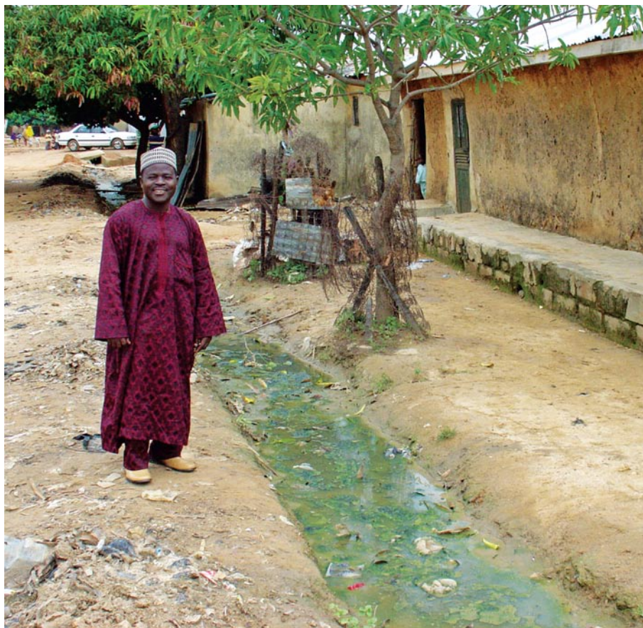
Figure 1. A drainage canal constructed by local community efforts in Zaria City, Nigeria, a malaria region. Dr. Samaila U. Dakyes, of the Department of Industrial Design, Ahmadu Bello University–Zaria, is a local chief who has organized people in his community to maintain sewers and waste control. Such efforts can improve conditions, but the stagnant water shown in the photo indicates the need for additional work and infrastructure. Photo by S. Batterman.
